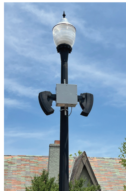
Basic Exposed Speaker Station
