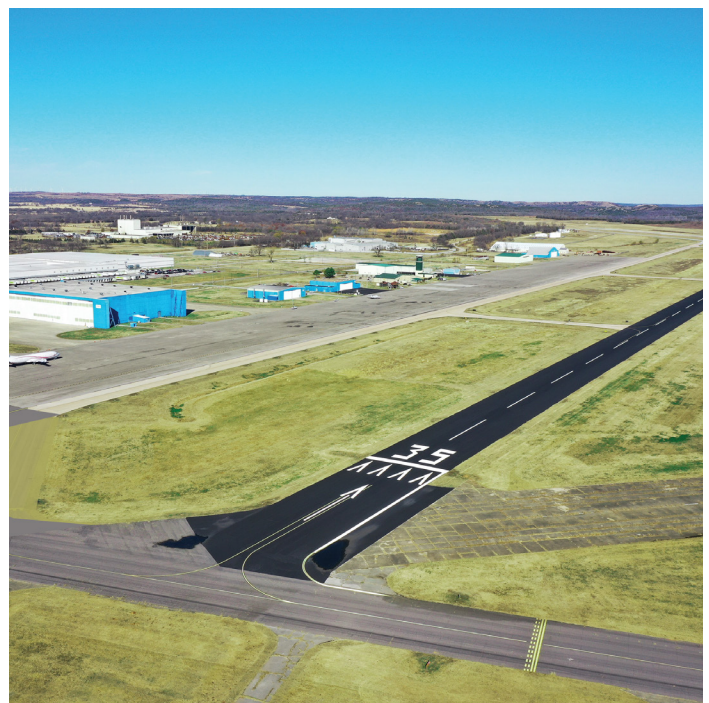
Ardmore Municipal Airport Realignment of Taxiway C
