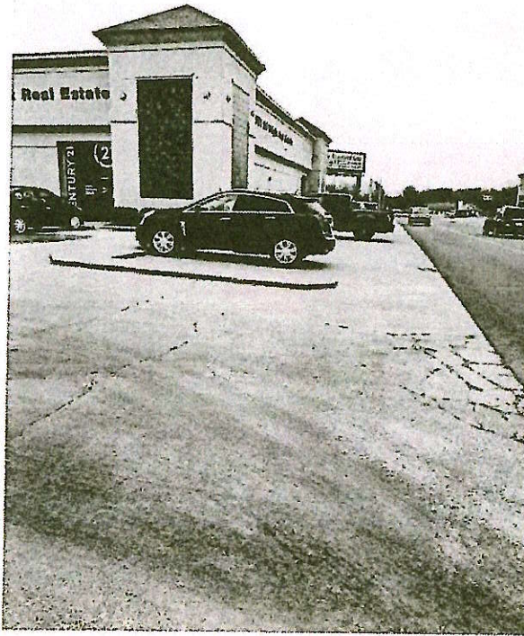
Examples of local businesses backing into street/right-of-way
